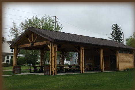
City Park Shelter Completed 2015
