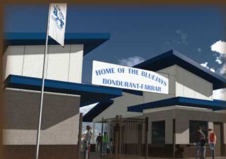
Bondurant-Farrar Football Stadium Completed 2014
